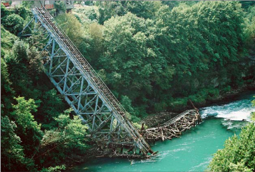
Bridge damaged in WWII © Ancient Land of Bosoni at en.wikipedia
