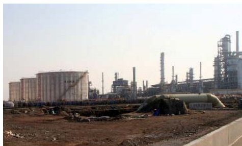
© Ryan Lackey Oil refinery and storage tanks
