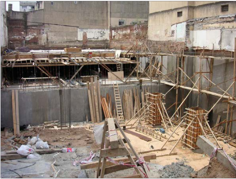
Construction site in Argentina © Beatrice Murch
